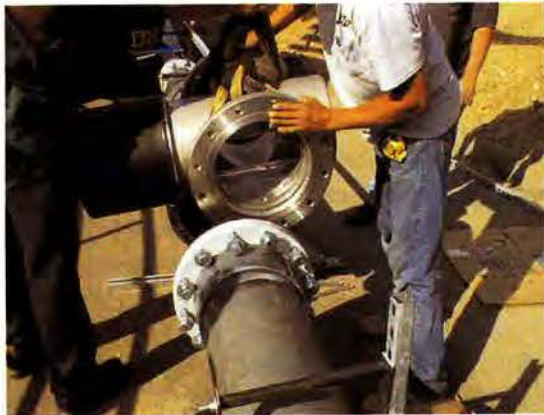
Figure 1. Installation of Trojan Technologies UVSwift 4L12 Unit
