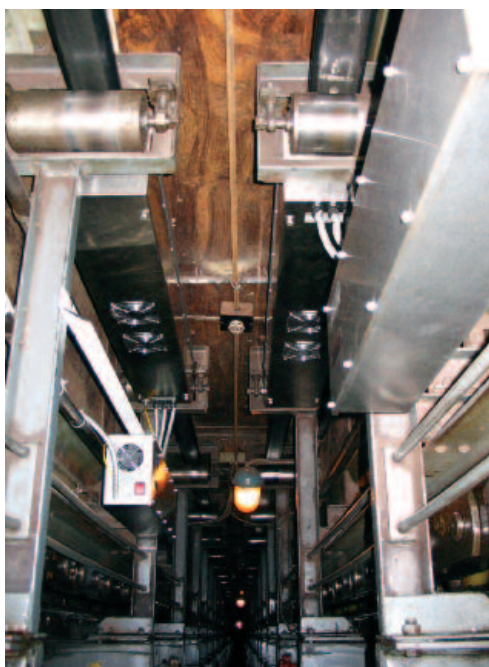
Figure 8. UV system mounted on a handrail return stretch at the "Kitai-Gorod" metro station.
